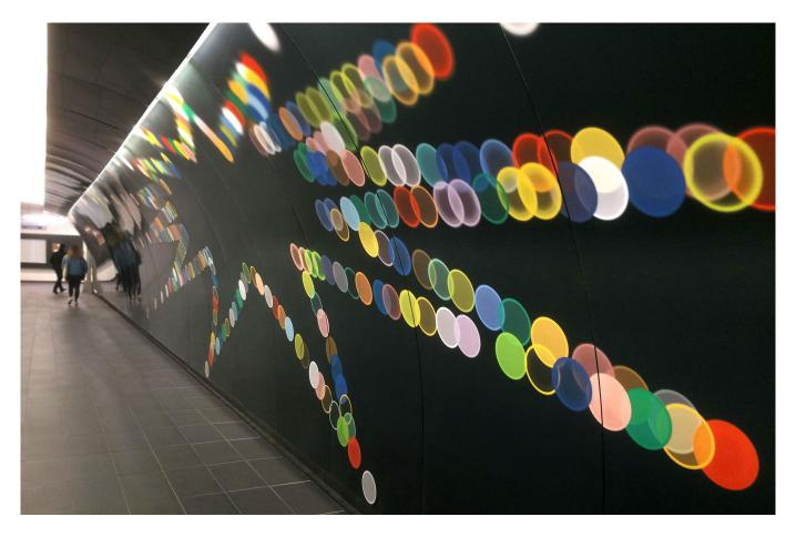
More durable than glass and just as beautiful, vitreous enamel, also known as porcelain enamel, offers a non-porous, glass-like finish created by fusing finely ground colored glass to a substrate through a firing process. Adding to its strength and durability, the substrate used is always a metal, whether precious or non-precious, for its stability and capacity to withstand the firing process.
